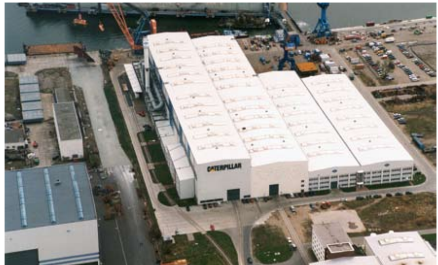
Picture: Caterpillar Motoren Rostock GmbH.
